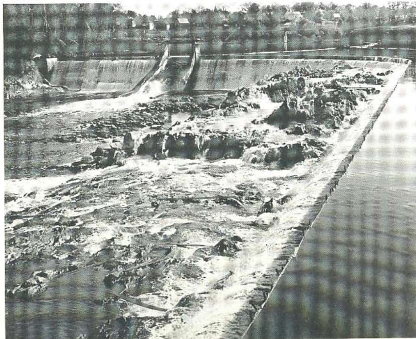
Lower Dam in Madison - Anson
